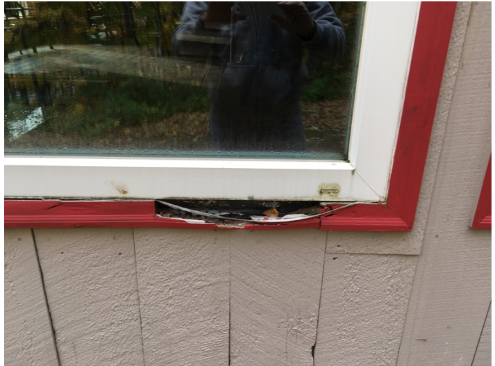
Figure 4. East Wall - Replace Window Sills.
