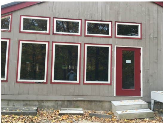
Figure 1. Replace East Wall - Add 1" Insulation.
