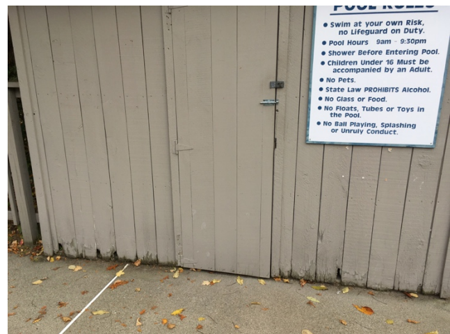
Figure 10. Replace Pool Shed Siding (2).
