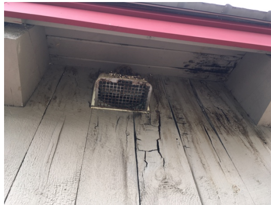
Figure 7. North Side - Repair Exhaust Fan Damage.
