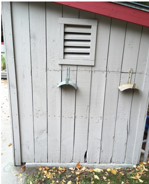
Figure 9. Replace Pool Shed Siding (1).
