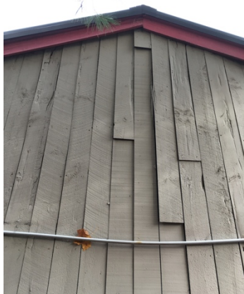
Figure 5. West Wall - Replace 20% of Siding & Add Eave.
