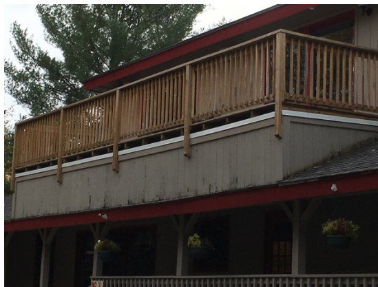
Figure 8. Replace Siding on Apartment Deck.
