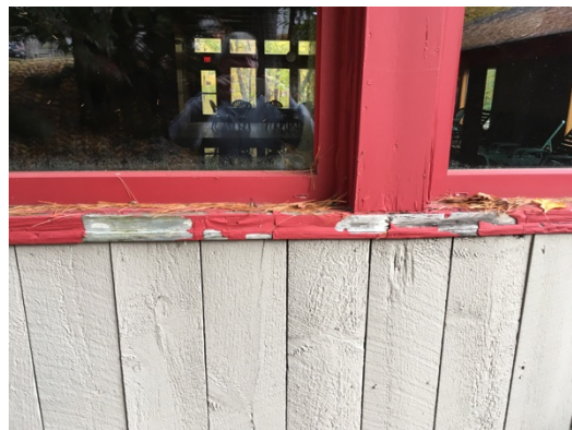
Figure 6. West Wall - Replace Window Sills.
